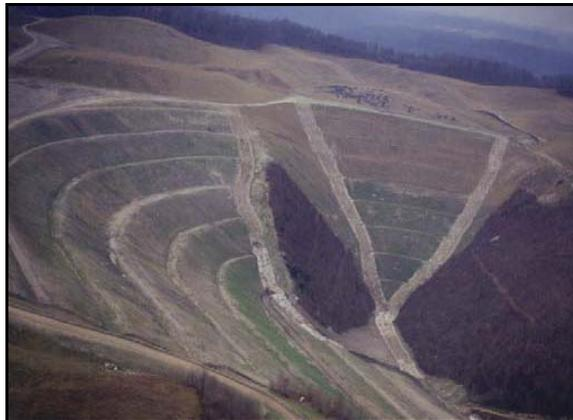
Figure 6: Comparison of concave (left) and flat (right) valley fill outslopes.
