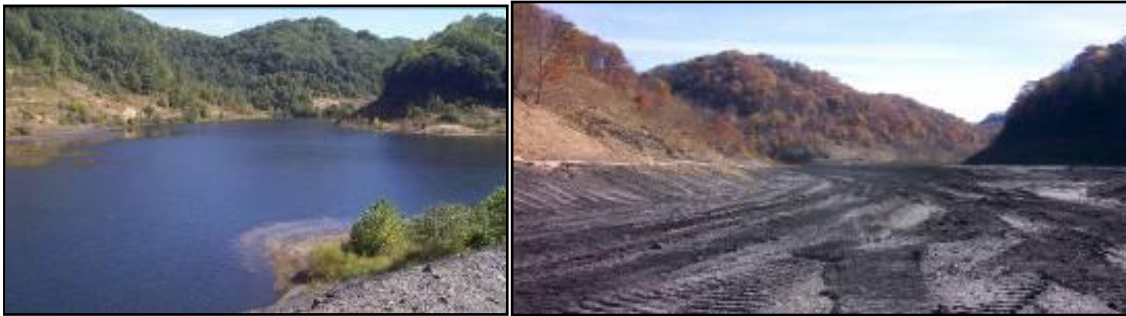
Figure 2: Pool of clear water above settled fine refuse prior to dewatering (left) and dewatered fine refuse (right) (modified from Shinavski, 2006).
