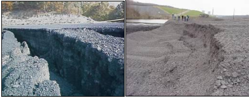
Figure 7: 1997 tension cracks (left) and 2000 slope failure in coarse refuse embankment of the Robena Slurry Impoundment in Masontown, PA (Smith et al., 2002).
