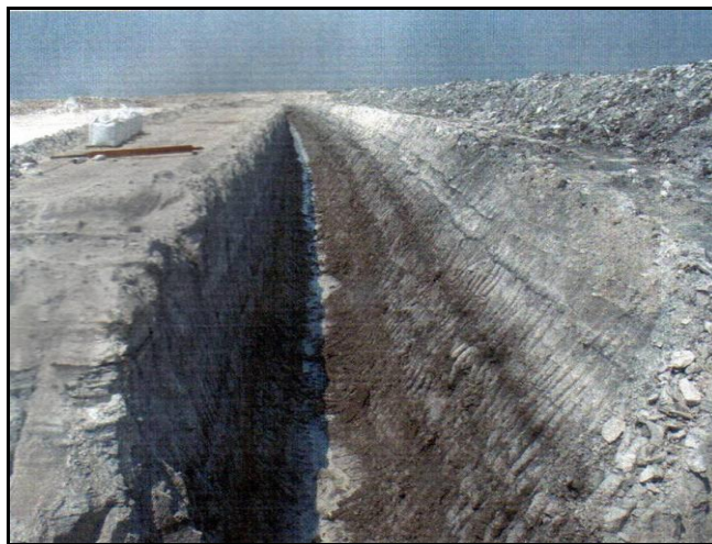
Figure 3: Dewatering ditch (modified from Shinavski, 2006).
