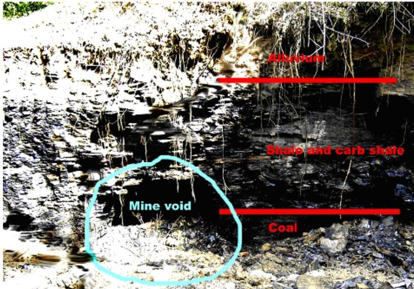
Figure 3 Exposed mine works and cover.
