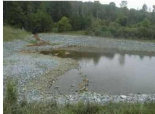
**This is a multi-cell passive treatment system, with the inlet on the left, and the water circulates through all the cells prior to discharging into the stream.**
