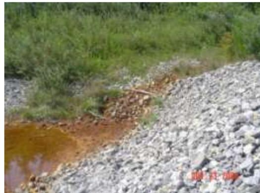
**The discharge enters the passive treatment system. Note the discharge inlet in the background.**
