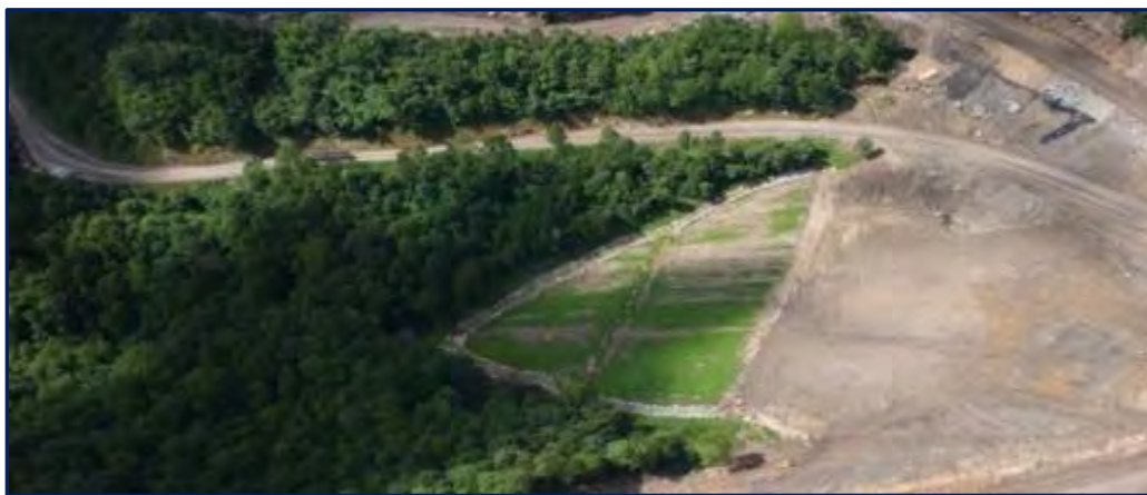
Aerial view of a hollowfill during construction
