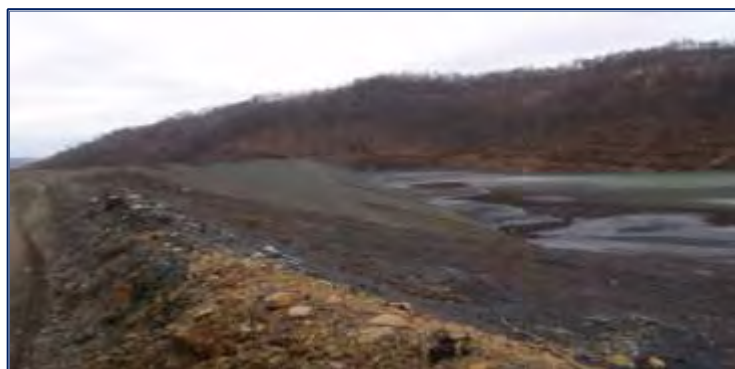
Slurry impoundment embankment
